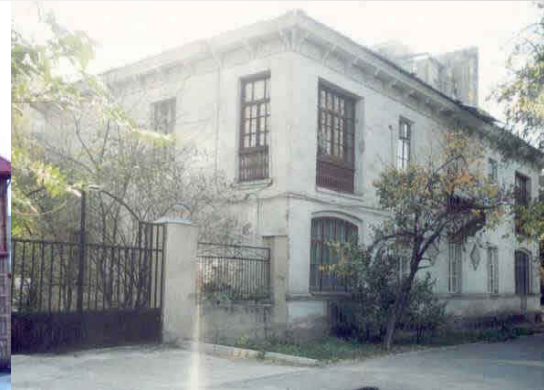
2story unreinforced brick masonry building with wooden floors
