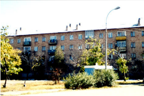
Buildings with hollow clay tile load-bearing walls and precast concrete floor slabs
